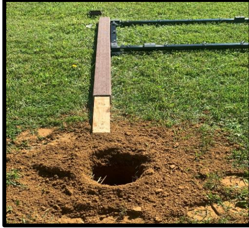
Dig post holes and Lift FREESTAND into place
