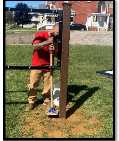
Backfill with concrete or gravel
